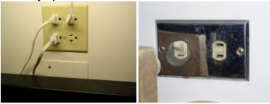
Ungrounded receptacle observed at right side of sink, recommend review by licensed electrician for corrections as needed prior to close.
